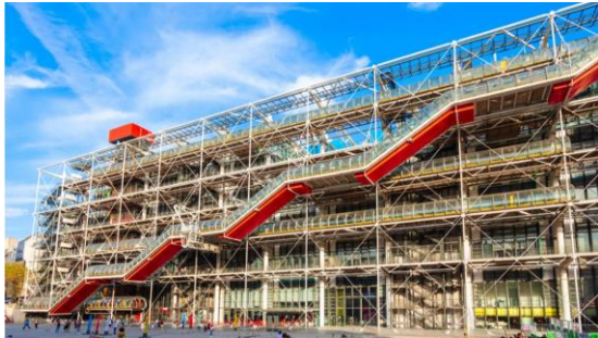
Gambar 5. Pompidou Centre, Paris
