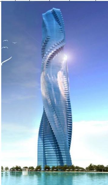
Gambar 9. Dynamic Building Dubai. Sumber : skyscrapercentre.com
