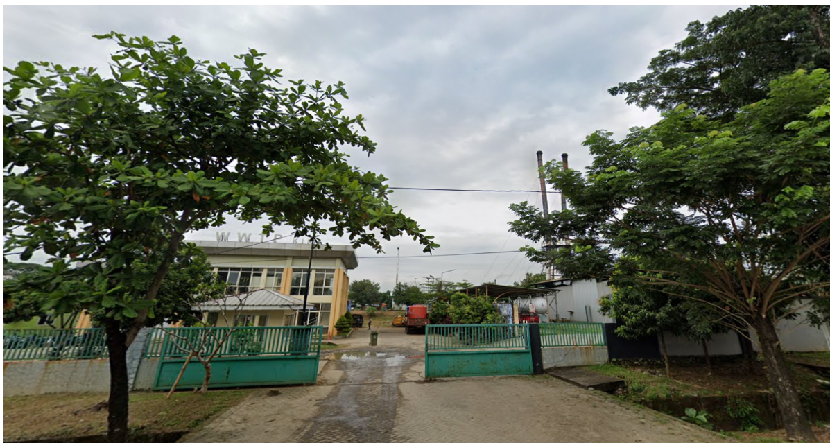
Figure 9. PT. KIMA Incinerator
