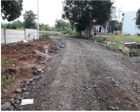
Picture 2. Project site facilities
