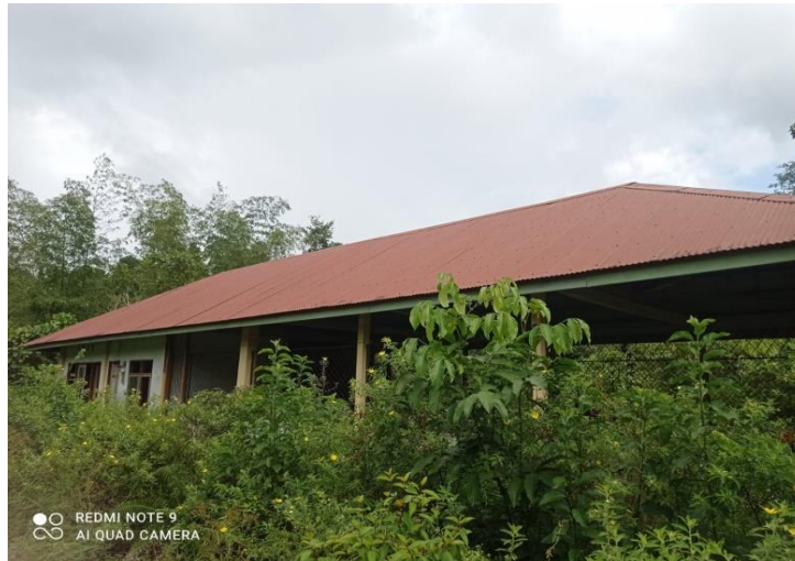
Figure 3. Abandoned waste warehouse in Simeulue Regency Source: processed by researchers (2023)
